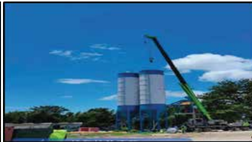
Installation of Batching Plant in Sitapur Sub Camp (SHIP)
