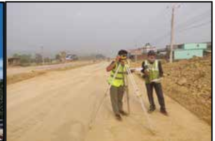
Level Checking of Embankment In NB Road (SRIP)
