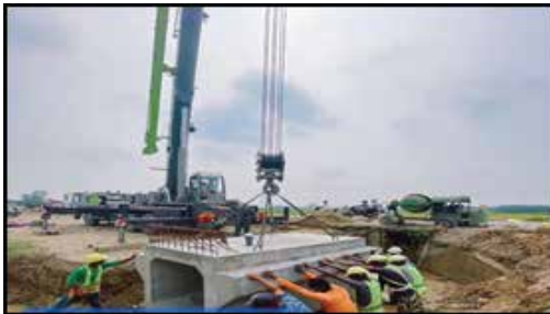
Installation of Pre-Cast RCC Box Culvert, Km 199+525 (SHIP)
